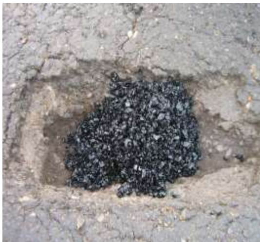
Fig. 2: Placement of Readymade pothole mix on NH206 Road
